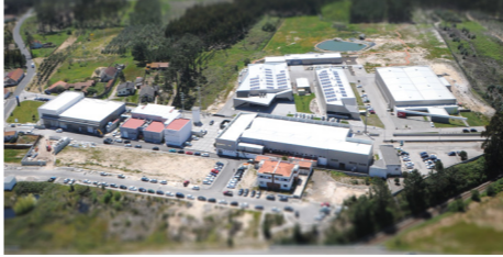
Grupo SOCEM Headquarters Tooling & Service Division – Martingança, Portugal
